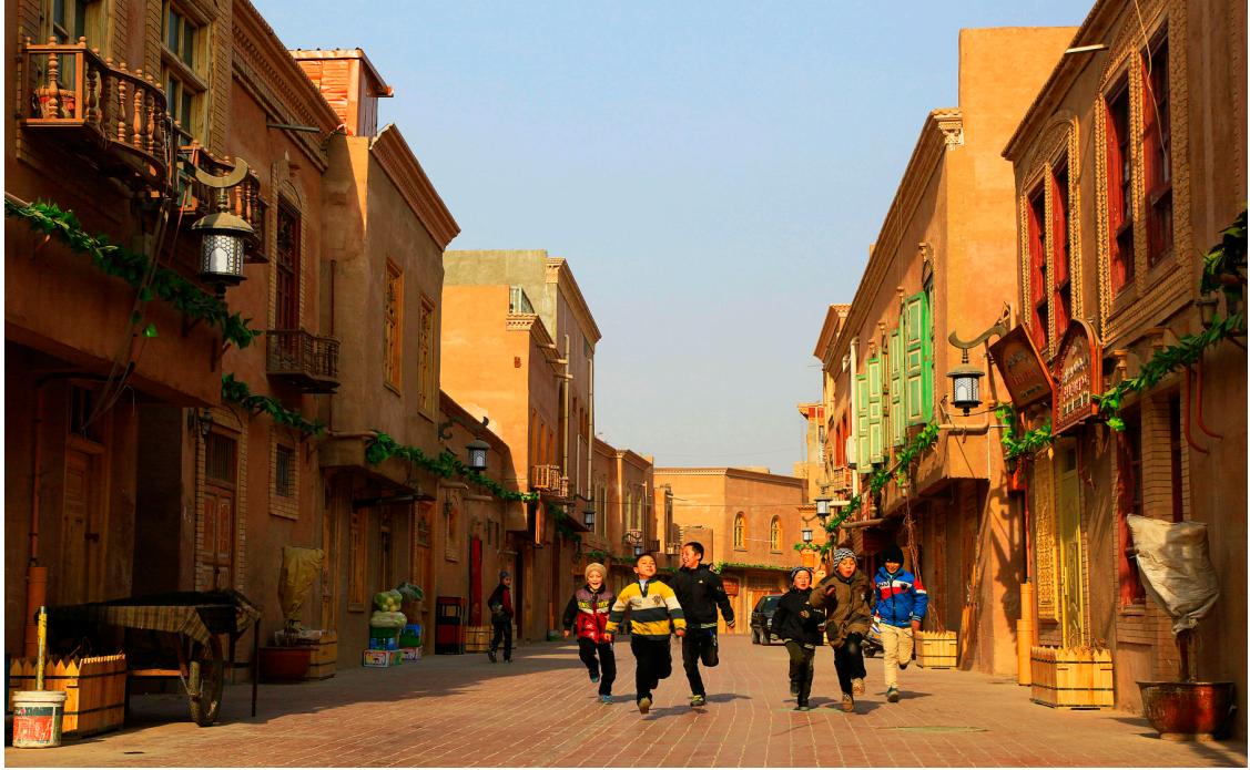
Figure 4.2.5 Different street views of traditional houses in Kashgar Old City (source: https://mehelle.biz )
