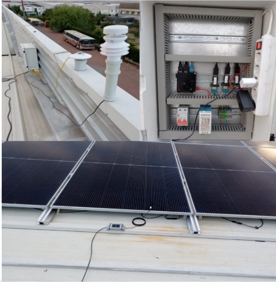
Figure 4.1 Sensors and Fisheye Camera Installation
