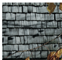
Timber facade cladding shakes
