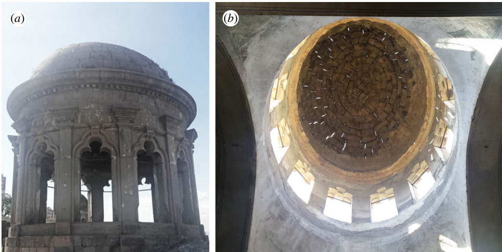
Figure 21. Oval dome of a run-down Orthodox church in Germin (Kayseri, Turkey). (a) External and (b) internal views. (Online version in colour.)
