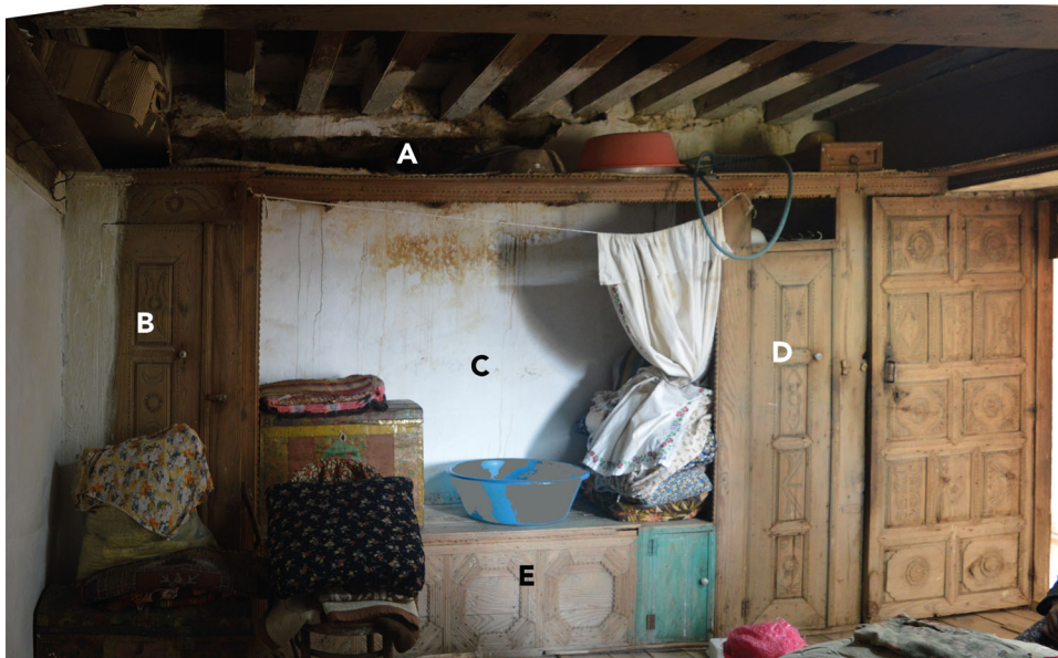
Figure 19. A. Pot shelf; B. Bathing cubicle; C. Closet; D. Display case; E. Pantry, abandoned house, Sarikaya village
