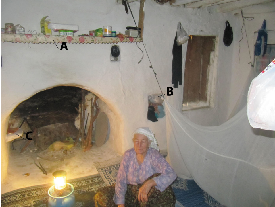
Figure 14. Fireplace. A. Fireplace shelf; B. Plate niche; C. Kindling shelf, İmpinar plateau
