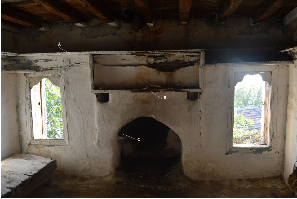
Figure 12. A. Upper shelf; B. Fireplace shelf; C. Kindling shelf, Türçen Karcıoğlu house, Sarıkaya village
