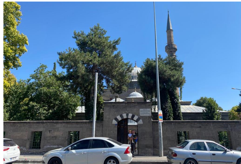
Figure 3.28 Kayseri Kurşunlu Mosque exterior space photos
