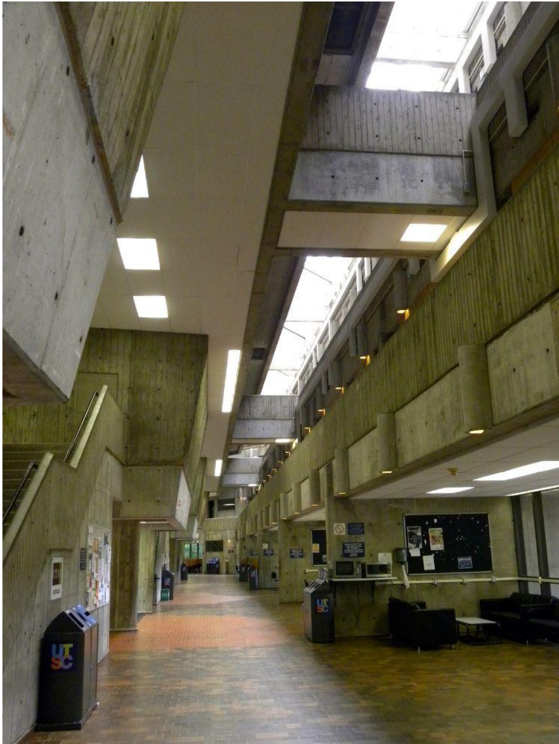
Figure 4-20 The Andrews Building in the University of Toronto Scarborough Campus, John Andrews, 1964-1966, Canada. (Photo courtesy: JasonParis. Flickr)
