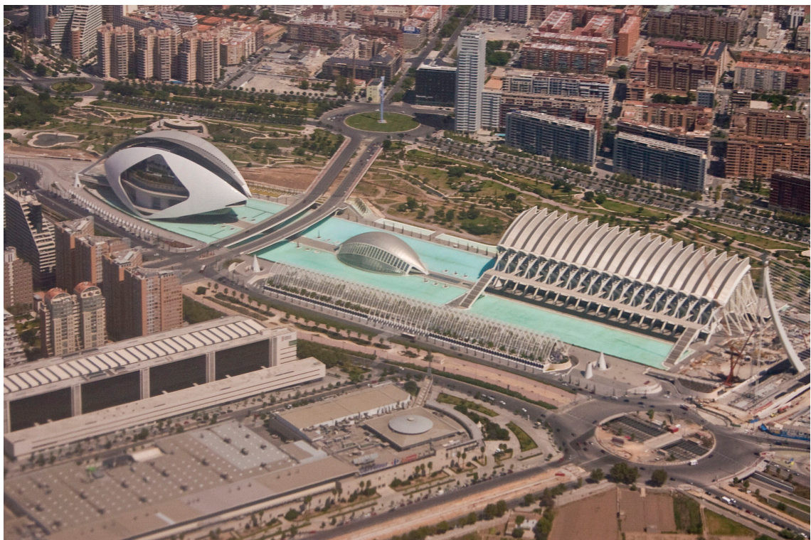
Figure 3-14 The City of Arts and Sciences, Santiago Calatrava and Félix Candela, 1996-2009, Valencia, Spain. (Photo: Mike Lowe)
