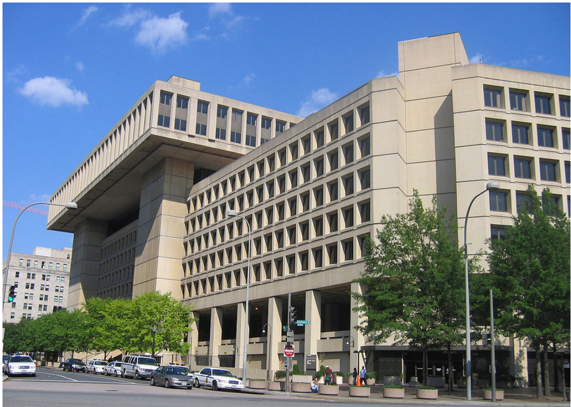
Figure 3-24 J. Edgar Hoover FBI Building, Charles F. Murphy & Associates, 1975, Washington DC, USA. (Photo: I. Aude)
