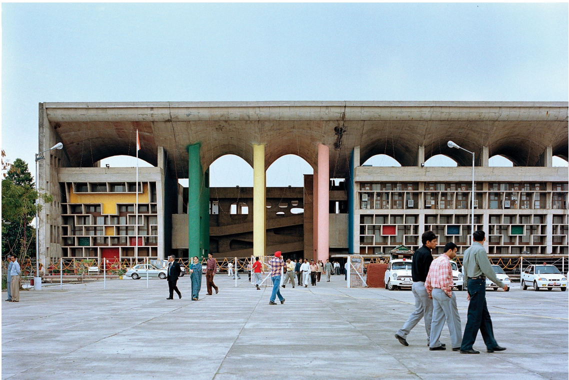
Figure 3-18 High Court Building, Le Corbusier, 1951-1964, Chandigarh, India. One of the three major elements in Chandigarh's Capitol Complex. (Photo: Bärbel Högner)
