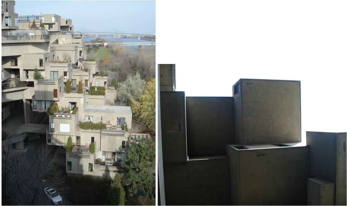
Figure 3-9 and Figure 3-10 Habitat 67, Moshe Safdie Architects, 1967, Montreal, Quebec, Canada. (Photos: Nilüfer Yöney, 2009)
