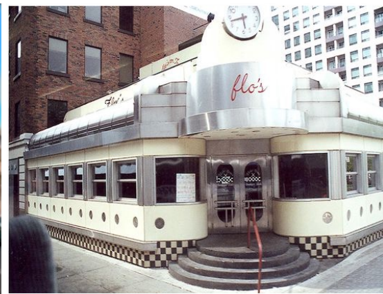
Figure 4-22 Streamline Art Deco dining car restaurant built in the mid-1980s, called initially 4D's Diner, later Flo's; demolished in 1998. (Source: woodsjesse, uglyhedgehog.com)
