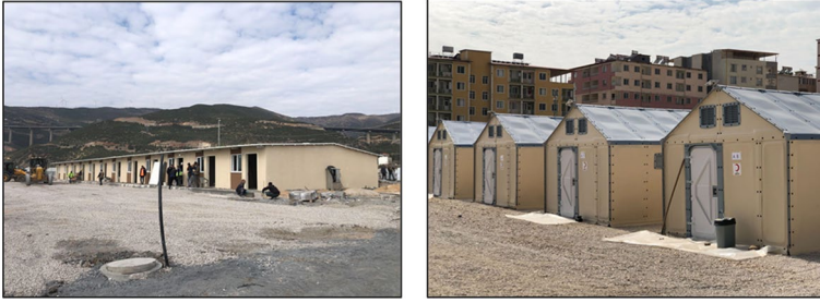
Fig. 8 Left: Temporary houses constructed by TOKİ in Nurdağı, Gaziantep; Right: Better Shelter Settlement in Hassa, Hatay (photographed by Nil Akdede and Özay Özaydın)
