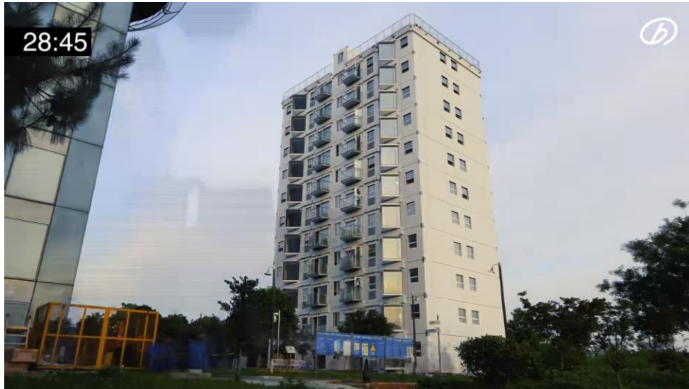
Figure 4.4.8 Ten floor stainless-steel modular building in 28 hours ( Ten-Storey Stainless-Steel Apartment Block Built in 28 Hours, n.d. )
