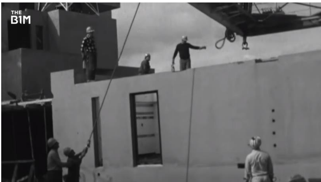
Figure 4.2.6 Workers during the construction of Habitat 67 (B1M, 2023)
