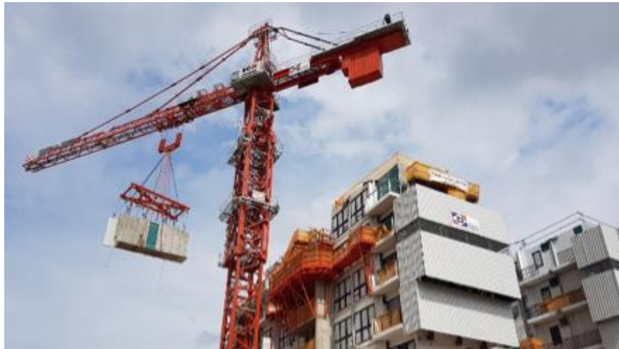
Figure 4.4.11 Tower Crane lifting a PPVC module ((BCA), n.d.)
