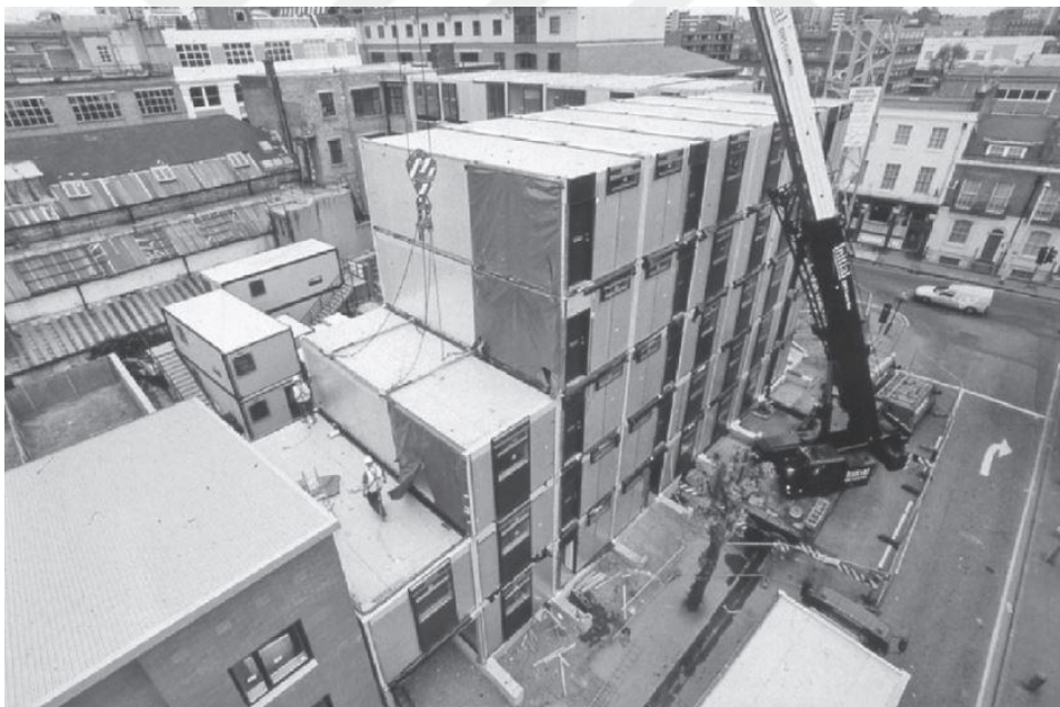
Figure 4.3.3 Murray Grove modules installation by crane (Lawson et al., 2014)
