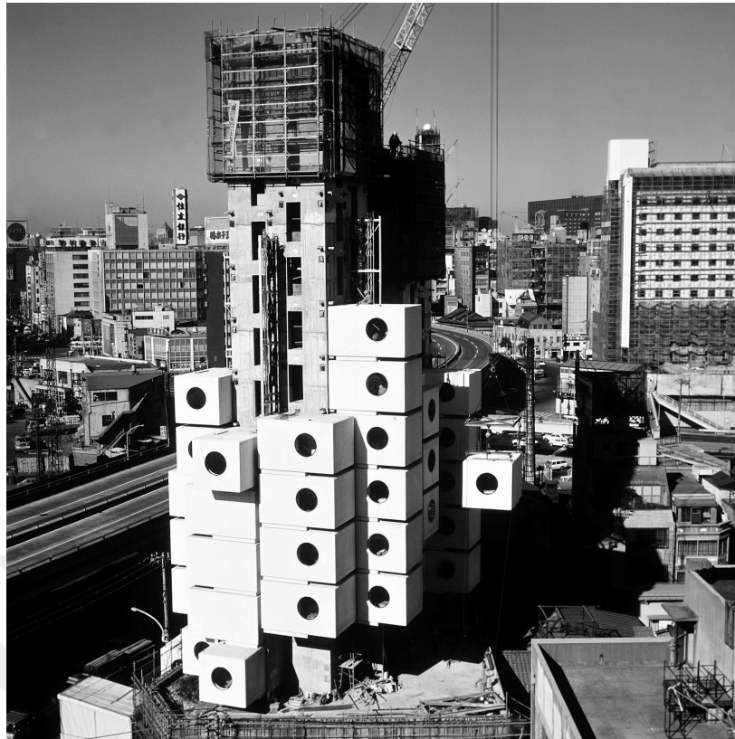
Figure 4.4.5 Nakagin Capsule Tower construction process (Lin, 2011)
