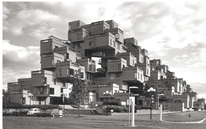
Figure 4.2.1 Habitat 67 historic view ( Habitat '67 , n.d.).
