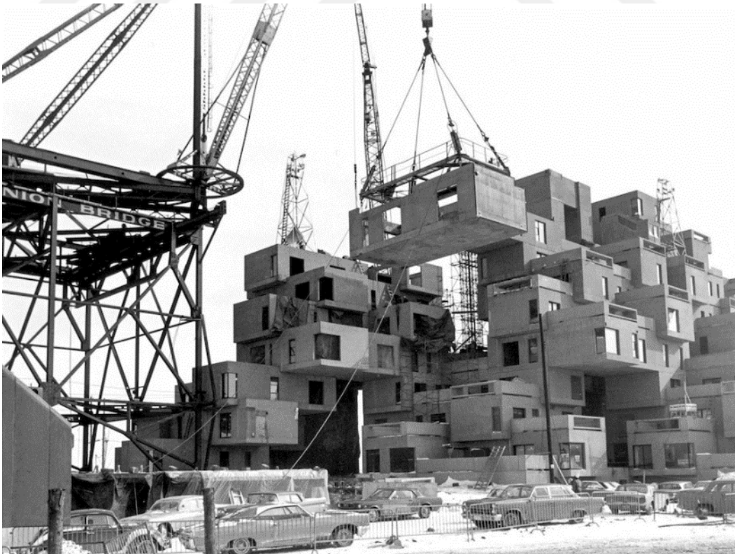
Figure 4.2.5 Lifting and stacking Habitat 67 modules by cranes ( Habitat '67 , n.d.)
