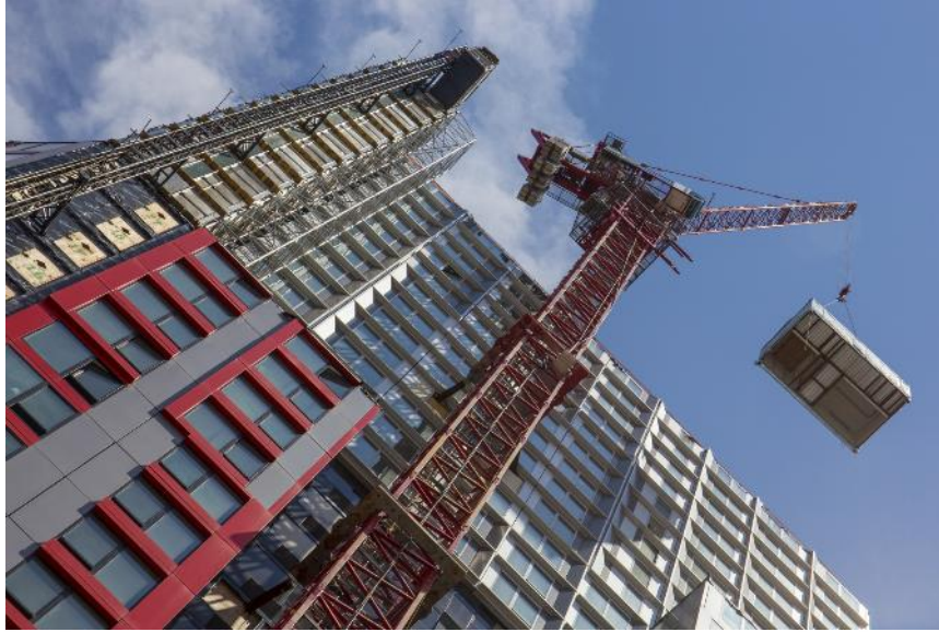
Figure 4.2.23 B2 Tower during construction, lifting a module by crane (B2 | SHoP, n.d.)
