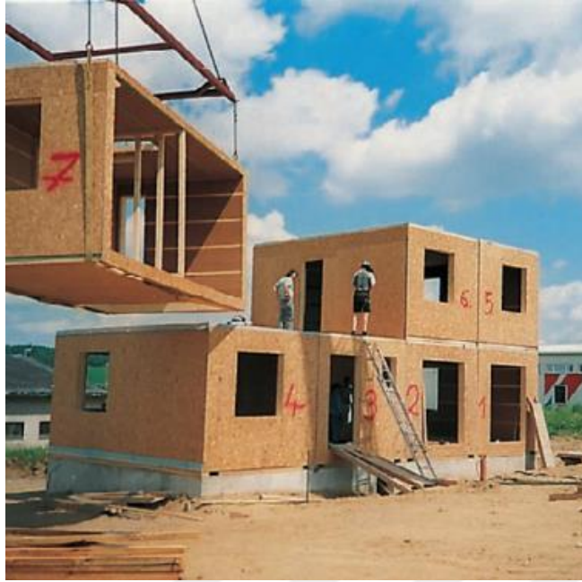
Figure 3.3.6 Timber module assembly process (Staib et al., 2008)
